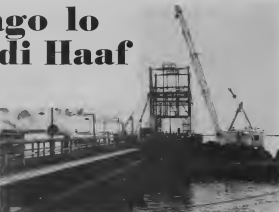
THE HOSE-HANDLING gantry, fabricated at Lago, was carried out on a barge and lifted into place by a floating crane. E STELLAGE di hoce, fabricá na Lago, a wordo trahá ariba un barge y poni na lugar door di un grua flotante.
